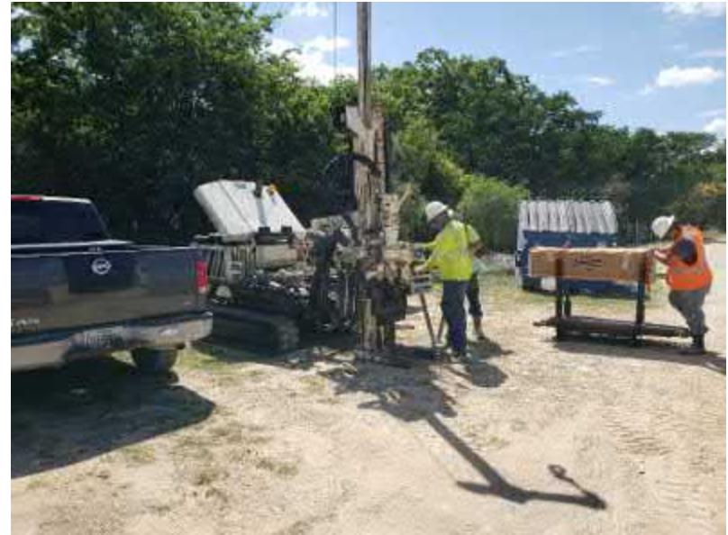
Photo #26 View of drill rig at soil boring B-15.
