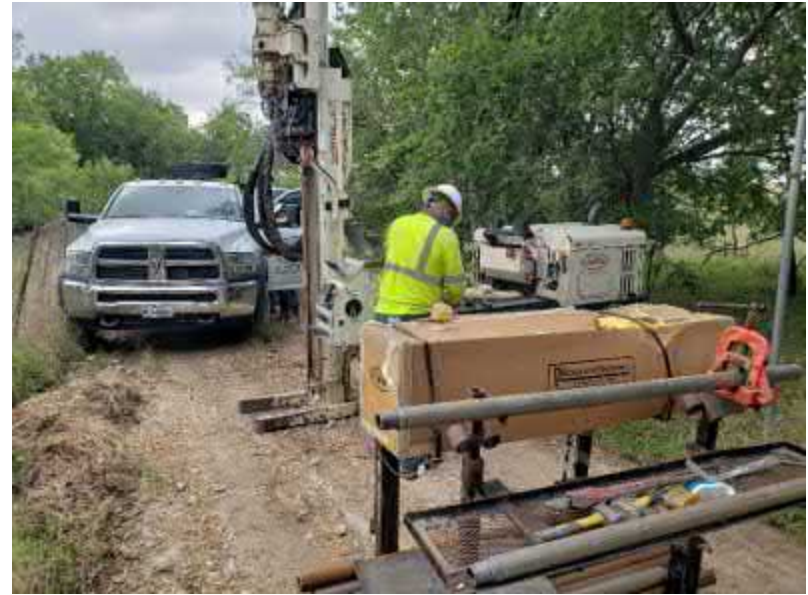
Photo #18 View of direct-push drill rig at soil boring B-7.
