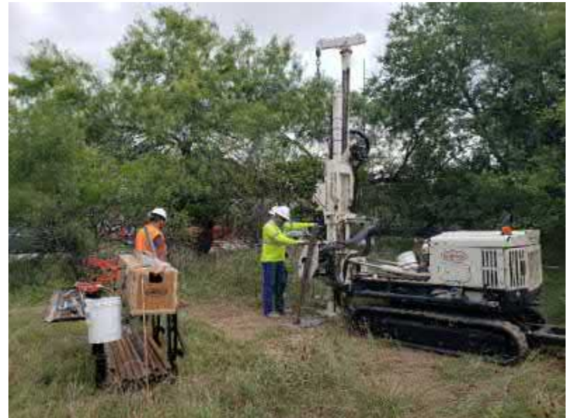
Photo #20 View of drilling activities at soil boring B-8.
