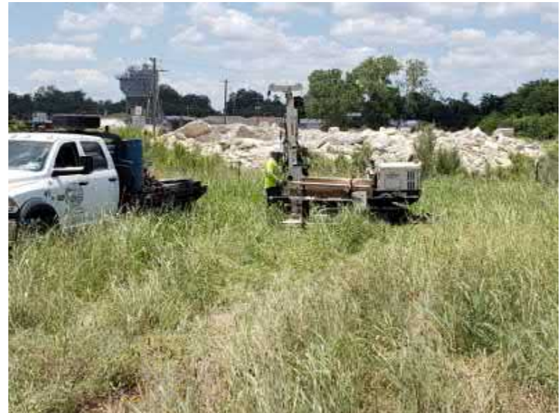
Photo #24 View of drill rig at soil boring B-13.
