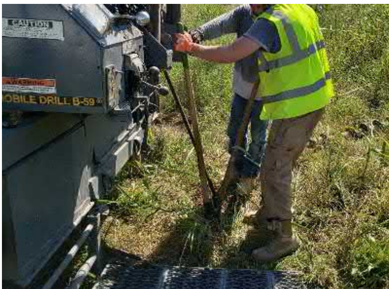
Photo #3 View of technicians excavating the upper few feet of the soil boring MM-2 using a post-hole digger.
