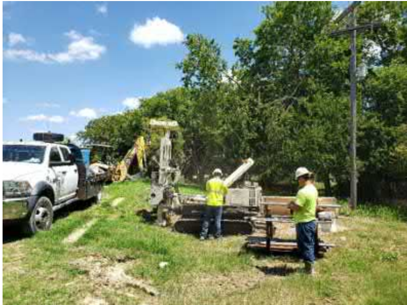
Photo #25 View of drill rig at soil boring B-14.
