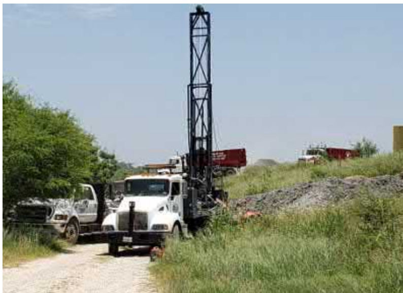
Photo #11 View of drill rig at soil boring location MM-4.
