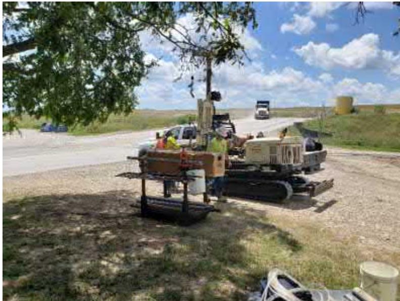
Photo #23 View of drill rig at the soil boring B-11.
