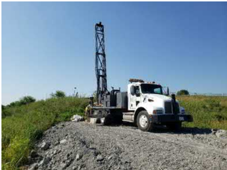
Photo #1 View of drill rig at location MM-1.
