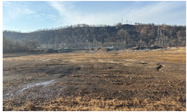
Photograph 2 : Site Overview Facing South
