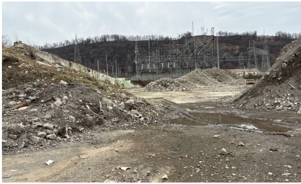
Photograph 1 : Site Overview Facing West
