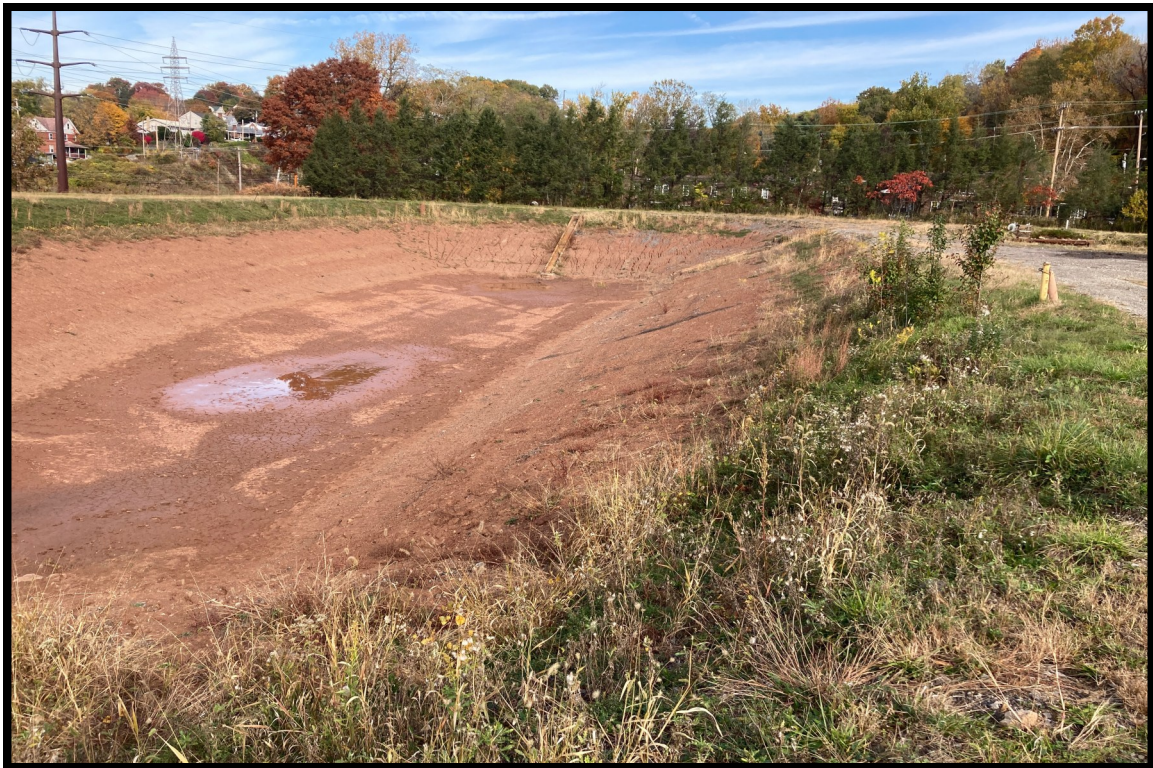
Photograph 2. Northern storm pond overview, facing northwest.
