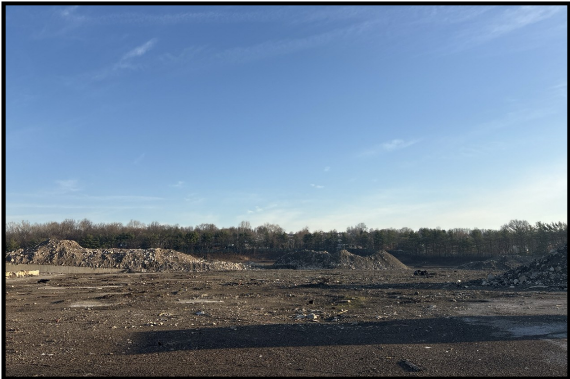
Photograph 8, Eastern project area, facing north.
