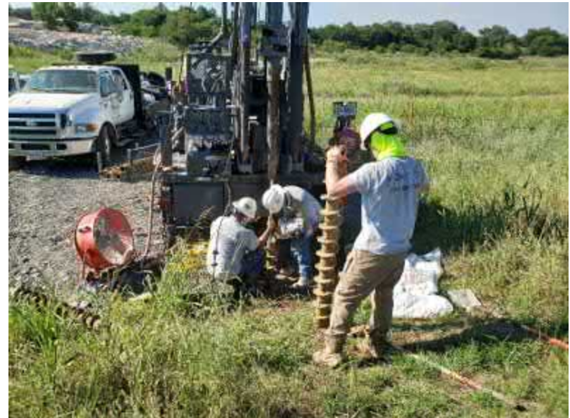
Photo #8 View of a drilling activities at soil boring location MM-3.
