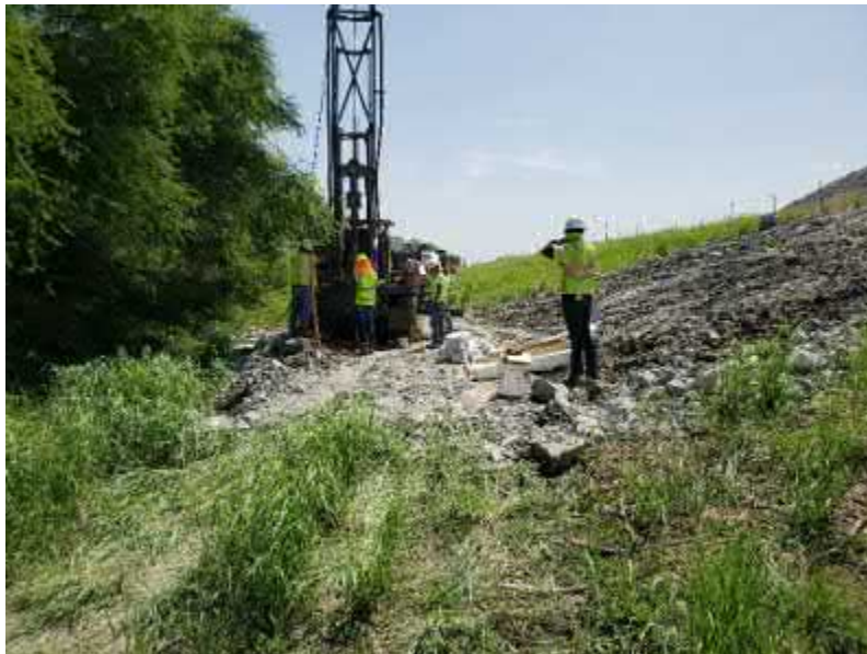
Photo #15 View of drill rig set up at soil boring MM-6.
