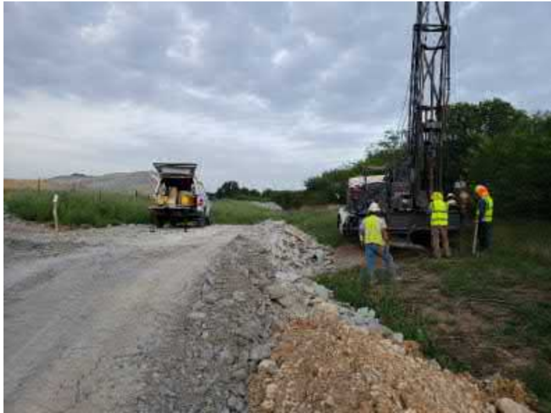
Photo #13 View of drill rig set up at soil boring MM-5.
