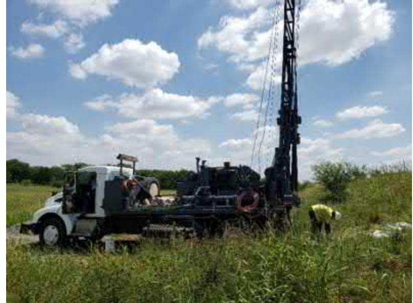
Photo #6 View of drill rig at location MM-2.
